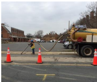
If debris is in the curb, a vacuum truck may be needed to clean up the area.
