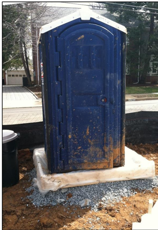
Portable toilet is located on level ground, and is inside secondary containment.
