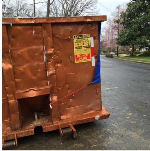
Good example of dumpster best practices. The dumpster is tarped and the tarp is secured. Traffic cones keep the area around the dumpster free of traffic and reflective tape (see bottom photo) is affixed to the ends of the dumpster.
