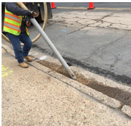
Example cleanup methods. Left photo: vacuuming. Right photo: sweeping debris away from the storm drain.
