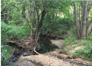
Existing stream bank erosion
